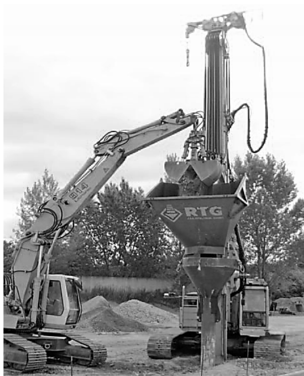
Figure 2. Filling the drilled well with soil and its compaction
